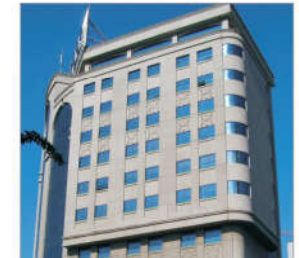
China Telecom (Beijing) Office Building Place: Beijing Area: 15000m 2 Panel Type: SC panel with HPL finish
